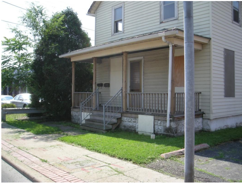
Grass cut and debris picked up
