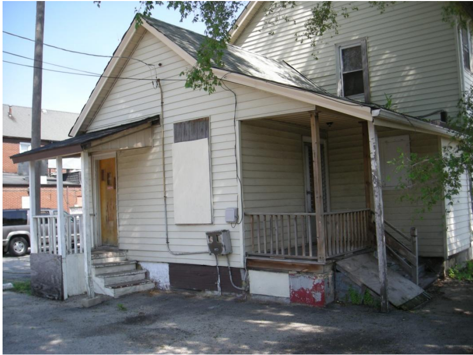
West elevation and south entrance to second floor unit
